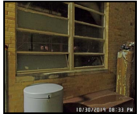
Windows open boiler area High School
