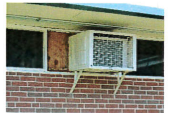
Typical Window Air Conditioning Unit
