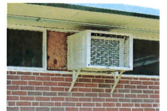
Typical Window Air Conditioning Unit
