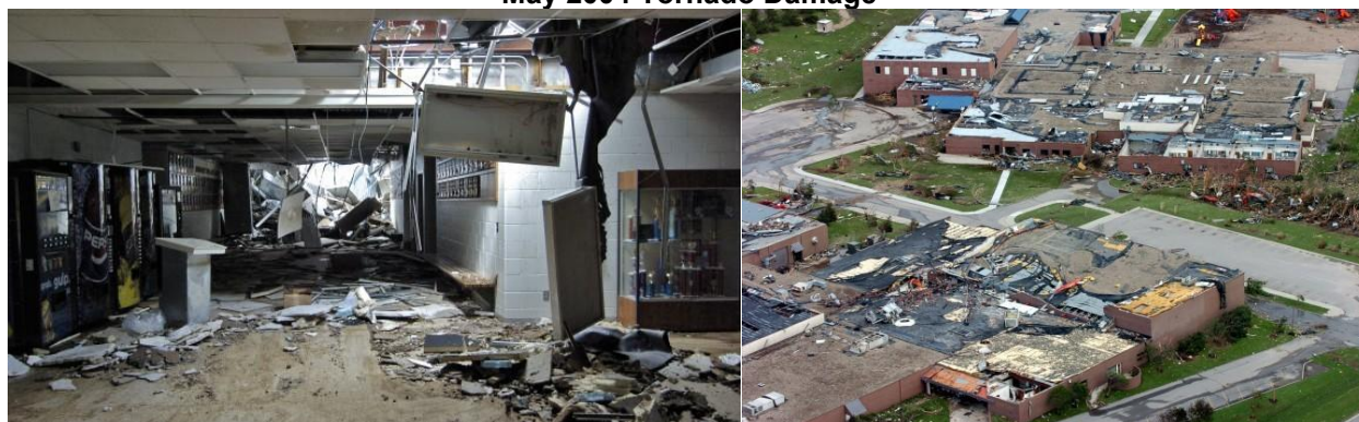
May 2004 Tornado Damage
