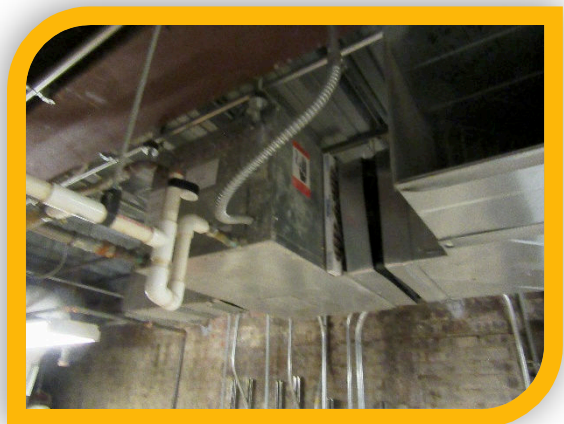
Water Source Heat Pump
