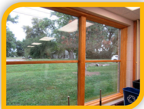
New Classroom Windows
