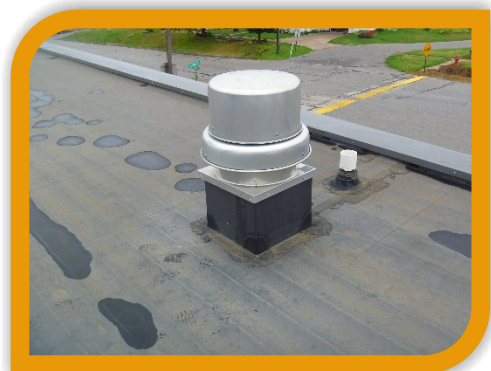
Powered Exhaust Fan
