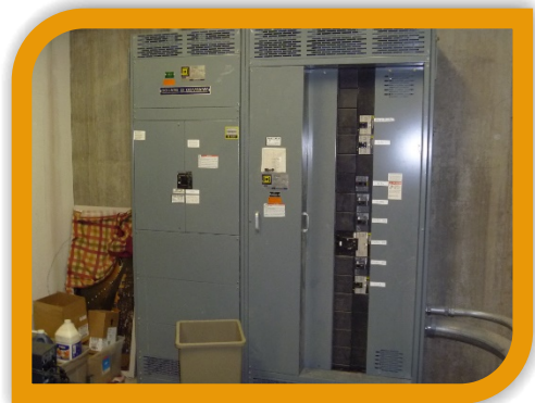
Main Electrical Distribution Panel
