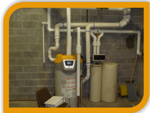
Heat Pump Boiler
