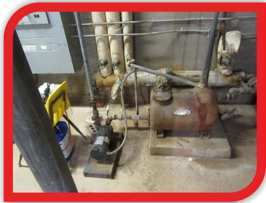
Steam Condensate Receiver
