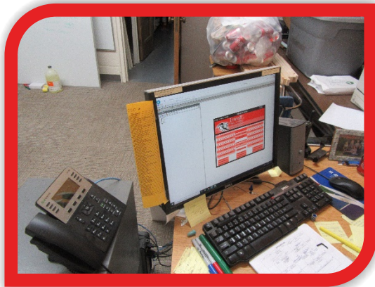
Building Automation System
