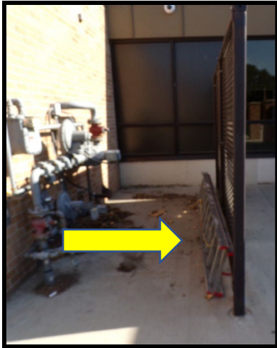
Ladder by door 4 area
