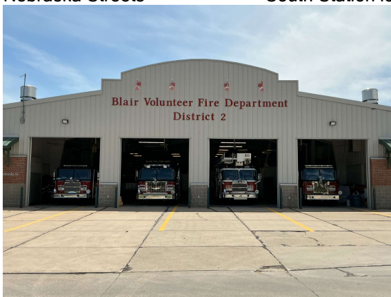
North Station located at 19 th and Nebraska Streets
