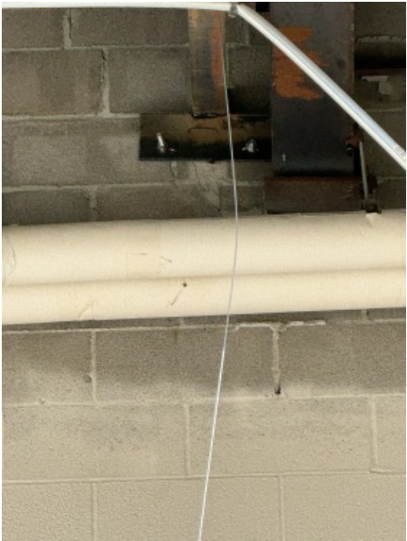
Support steel supporting the North CMU wall which will stay.
