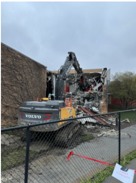
Started to take down the Blue Gym building on 4/1
