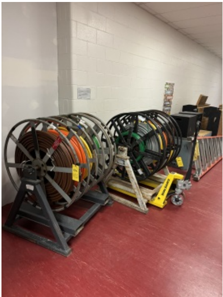
Wire Spools ready to be pulled into the pump room.
