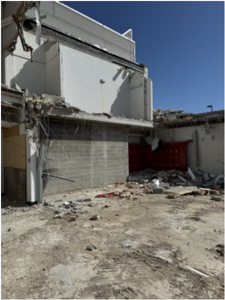
North Wall in the old locker room area.
