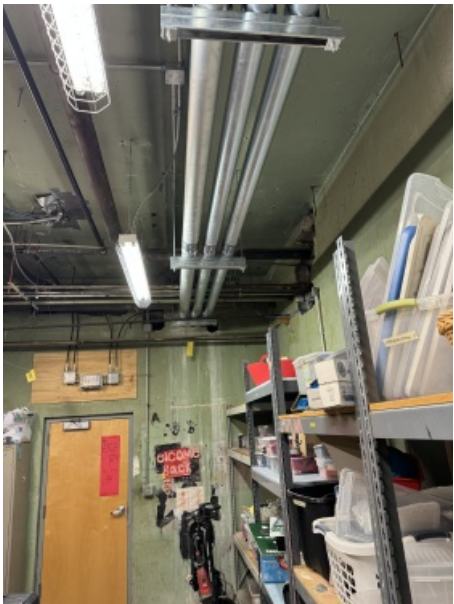
Conduits routing towards Activity Gym.
