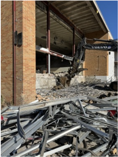
Taking out the steps into Pool area.
