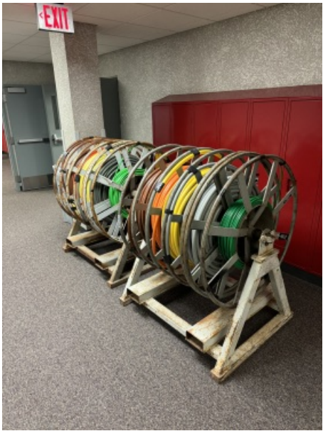
Wire Spools ready for pulling on Saturday.
