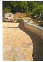
CONCRETE SEAT WALL
