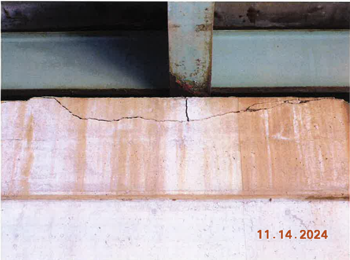
N face of Pier #6 at Girder #4.
