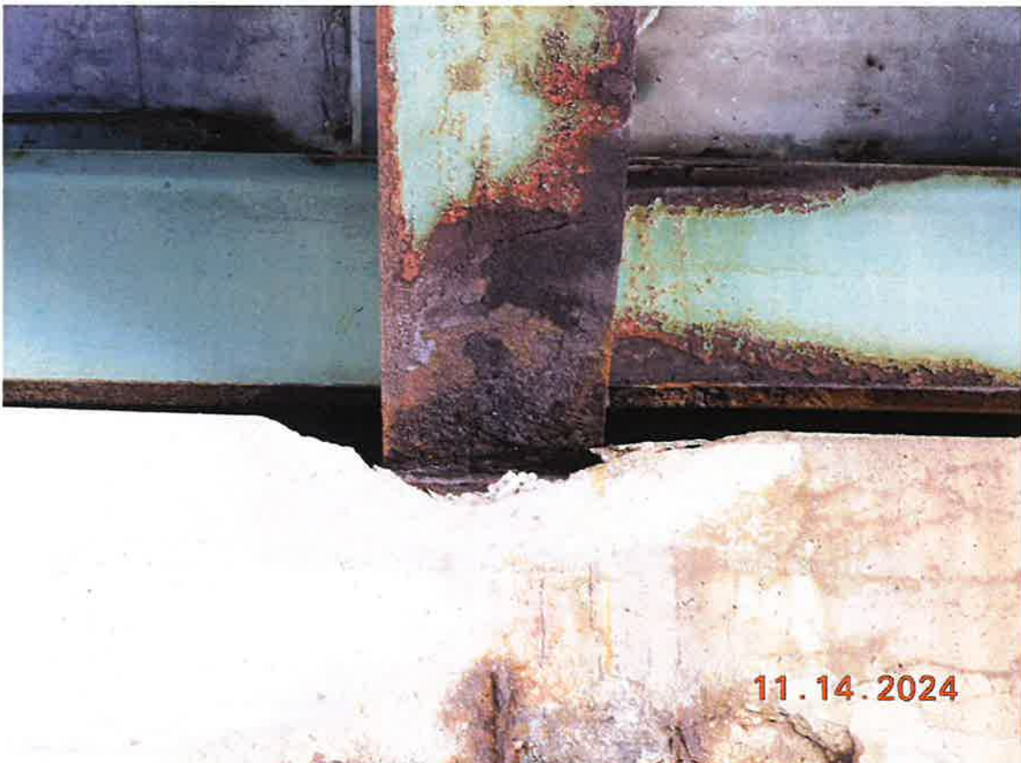
N face of Pier #6 at Girder # 6.
