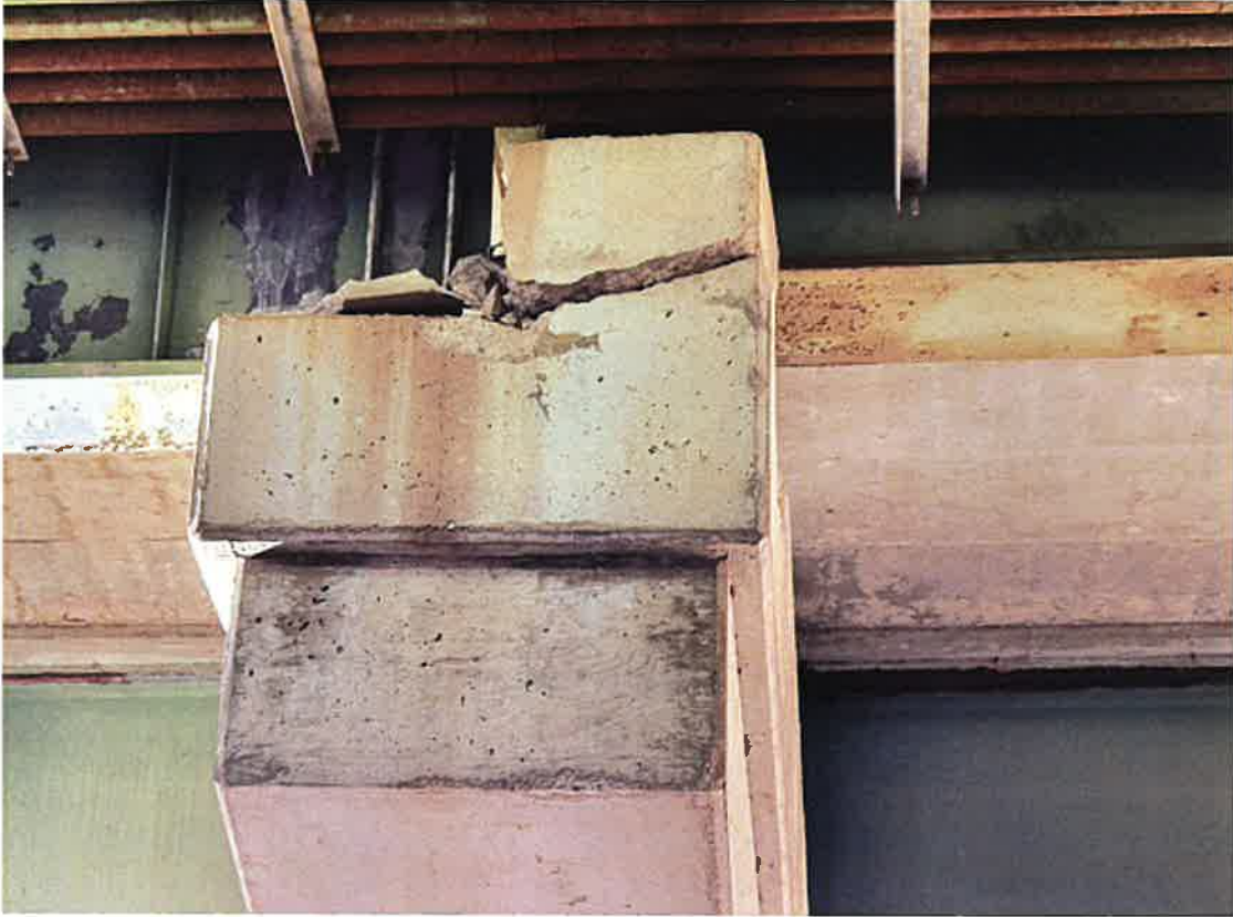
East end of Pier #6 cap.
