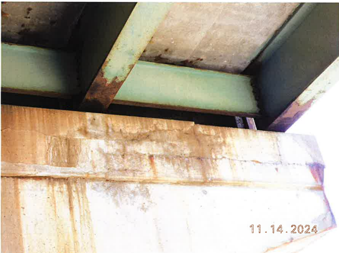
N face of Pier #6 at Girders #2 and #1.
