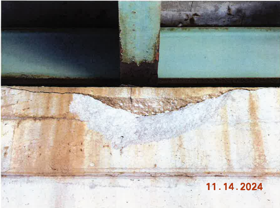
N face of Pier #6 at Girder #5.
