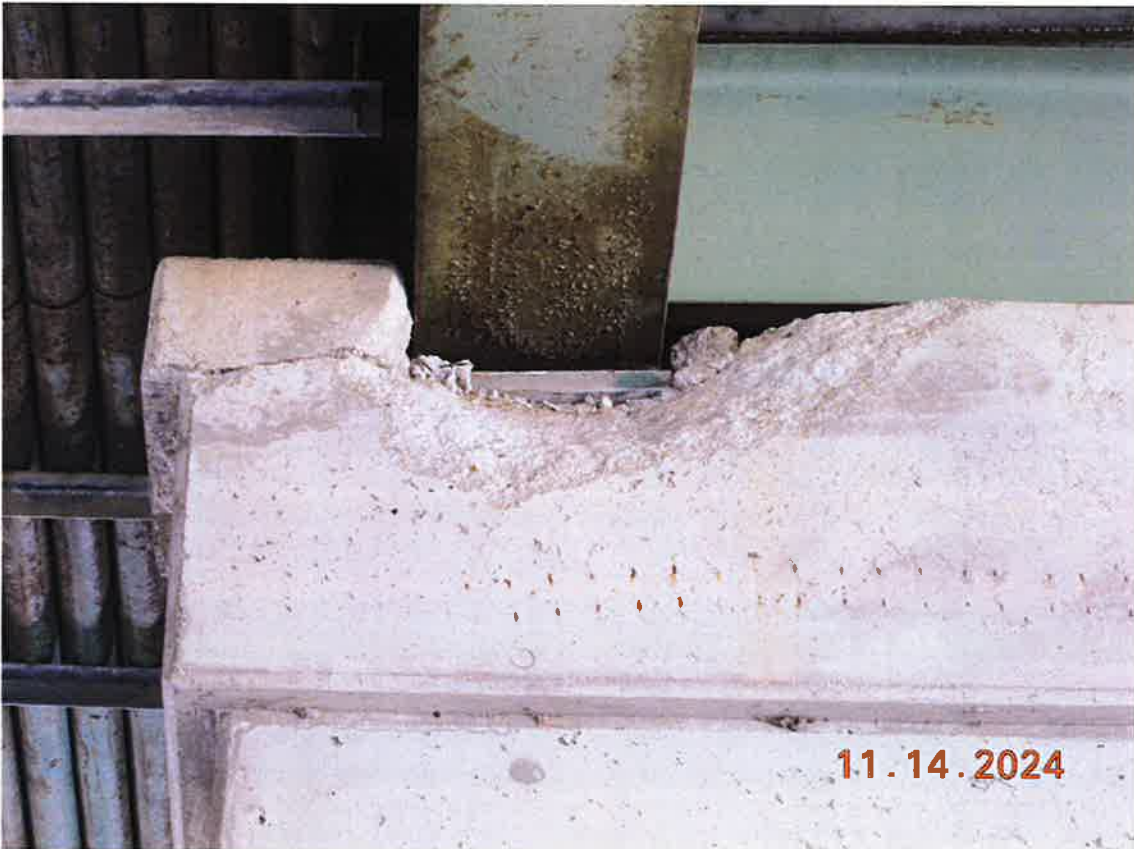
N face of Pier #6. Closeup of bearing area for Girder #7.
