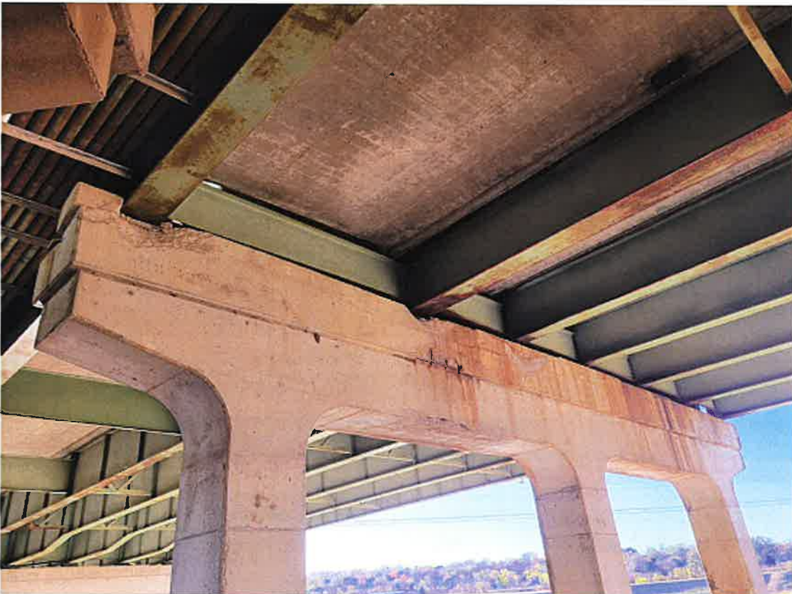
Far side of Pier #6 Cap.
