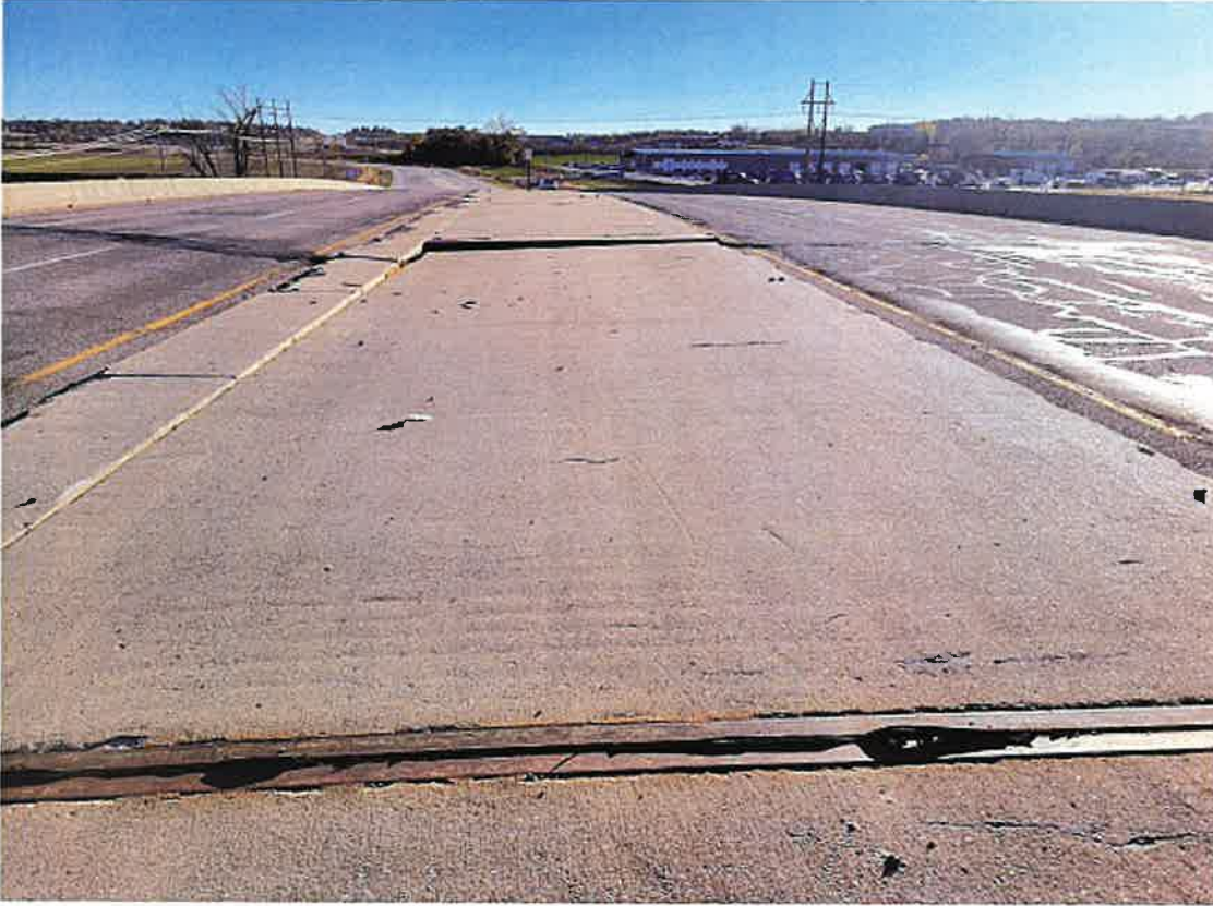
Looking south across Span #7 on the median.
