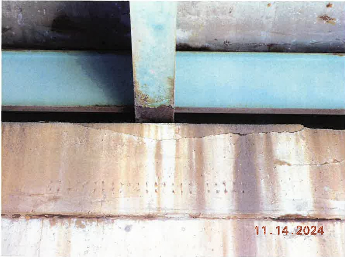
N face of Pier #6 at Girder #3.
