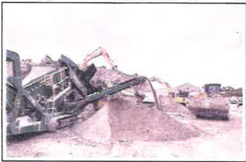
View 2: Crushing Operation
