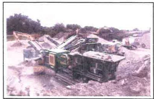
View 3: Crushing Operation
