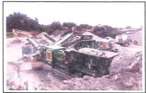
View 3: Crushing Operation
