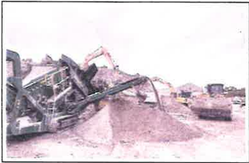
View 2: Crushing Operation
