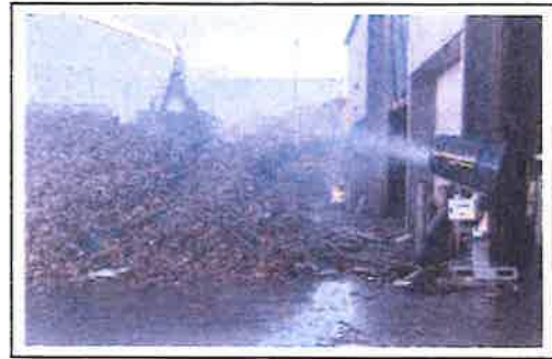
View 5: Screenpod S45 Dust Cannon in Operation
