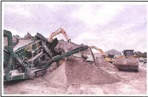
View 2: Crushing Operation
