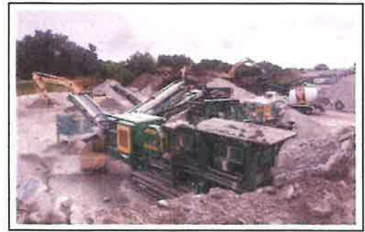
View 3: Crushing Operation
