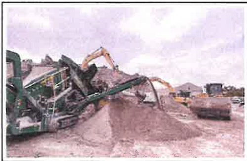
View 2: Crushing Operation
