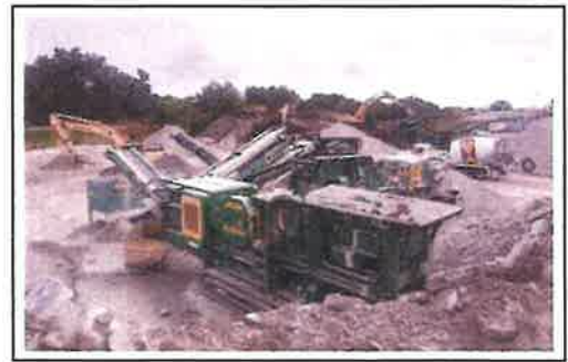
View 3: Crushing Operation
