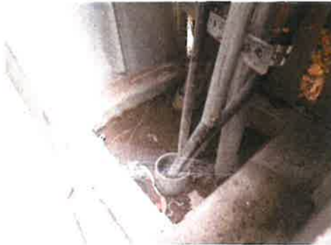
COAX PORT INSIDE ENCLOSURE SCALE: NTS
