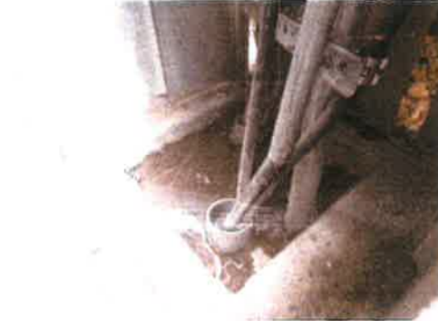
COAX PORT INSIDE ENCLOSURE SCALE: NTS
