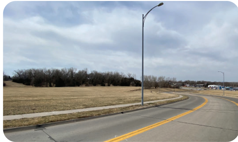
Looking west down Herman Drive toward Fort Crook Road
