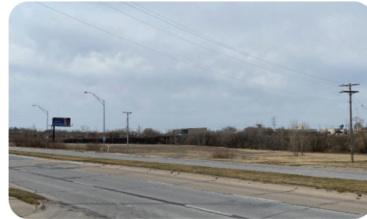
Large elevation change and wall delineates the site's south edge
