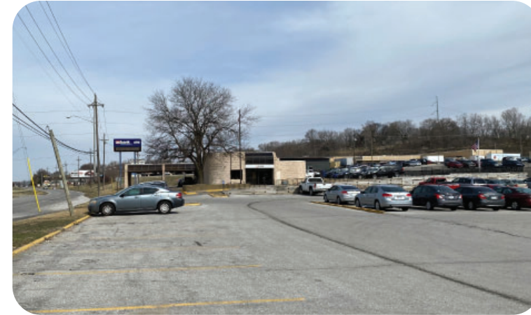
Utility lines and buildings mark the Fort Crook Road frontage
