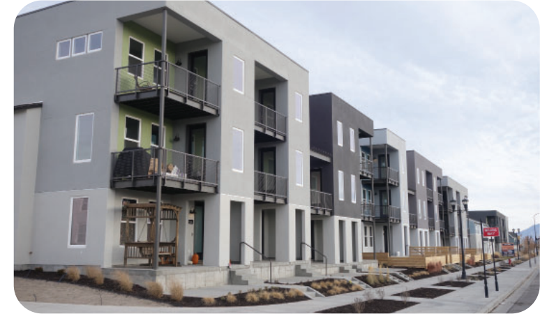
Multi-family residential building with a small, urban setback
