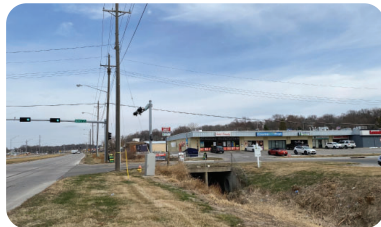
Looking north along Fort Crook Road at the Avery Road intersection
