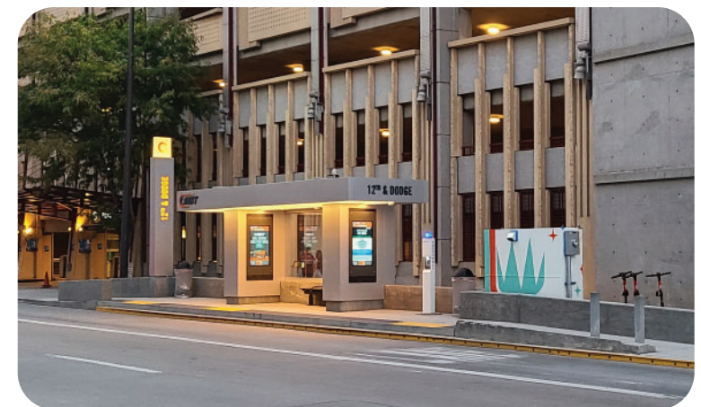
Existing Dodge Street ORBT station
