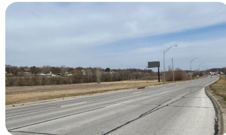
Looking north along Fort Crook Road with the cleared site off to the left
