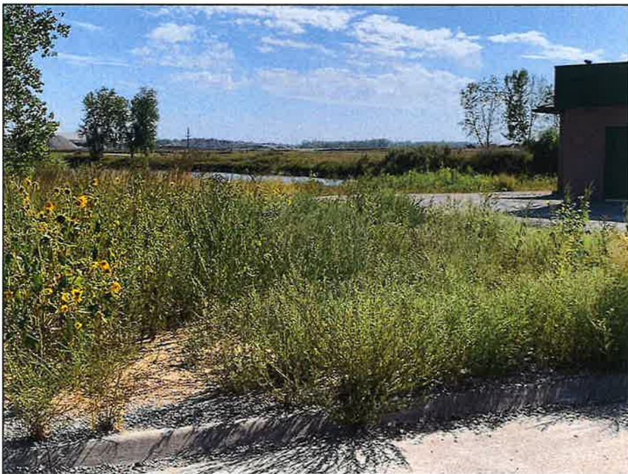
Looking south near existing lift station
