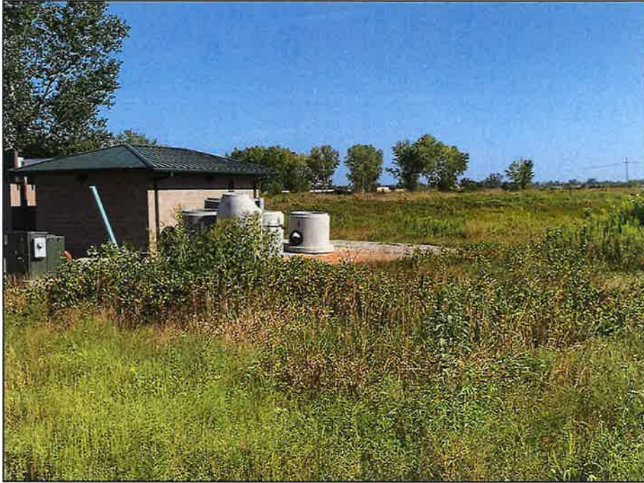
Looking southeast towards existing lift station
