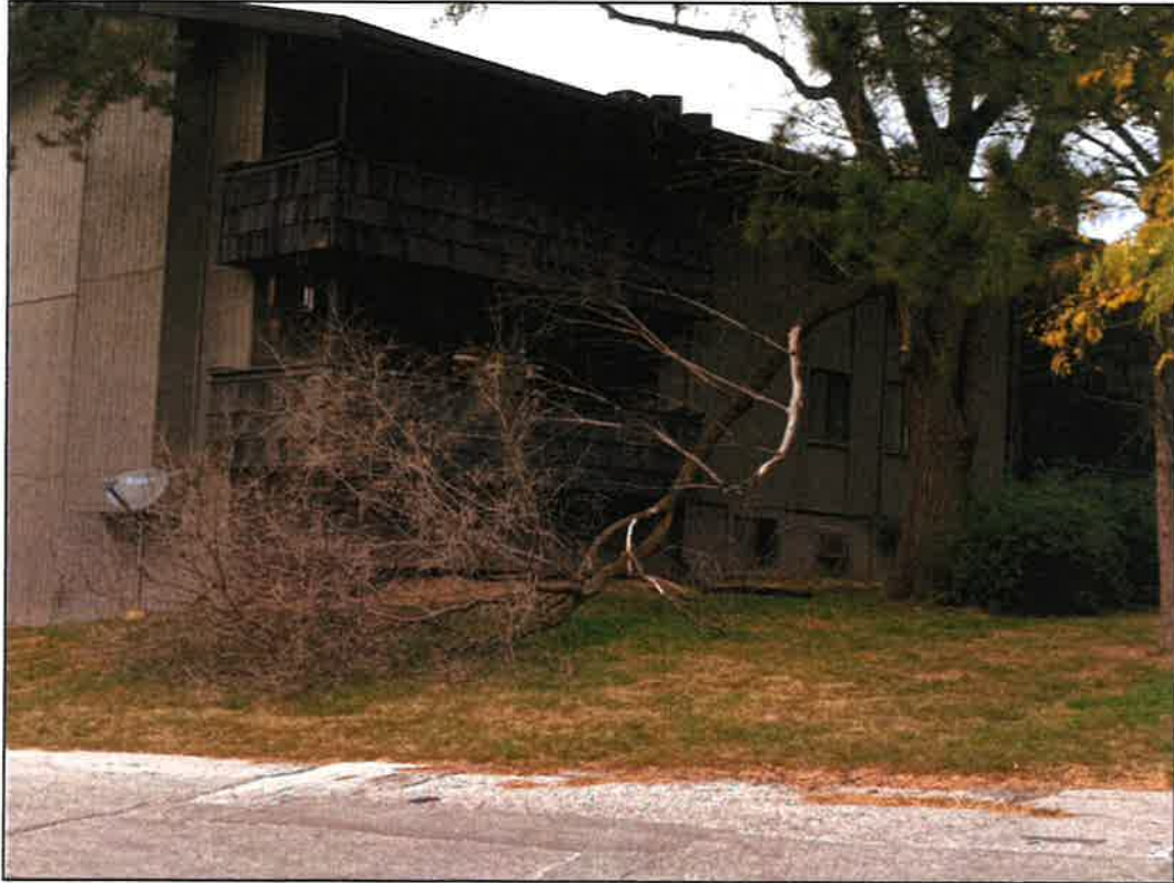
Storm debris remaining 10/20/21 after summer wind storm
