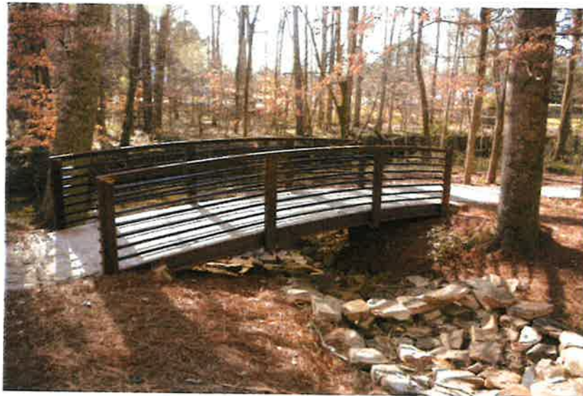
Figure 4- Steel Thru-Truss Bridge
