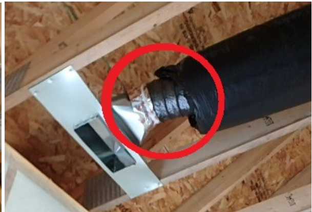
A “hybrid” spray-foamed metal & flex duct system . . . & register end of the flex.
