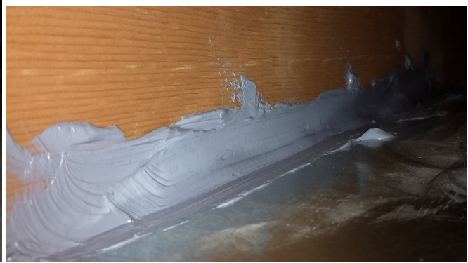
Unsealed metal RA Trunk to Joist connections are often unnoticed but add to leakage
