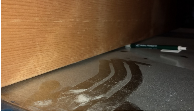
Unsealed metal RA Trunk to Joist connections are often unnoticed but add to leakage
