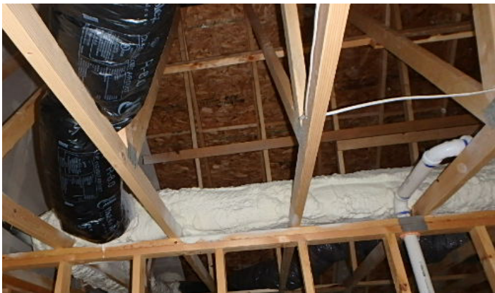
A “hybrid” spray-foamed metal & flex duct system . . . & register end of the flex.
