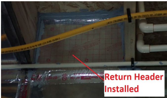
Missing RA Headers are often not noticed – but can create negative pressure zones that backdraft gas-fired Water Heater flues
