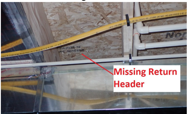
Missing RA Headers are often not noticed – but can create negative pressure zones that backdraft gas-fired Water Heater flues
