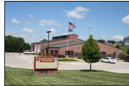
Photo B-31: District 4 Station
