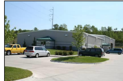
Photo B-33: Fire Training Facility
