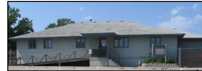
Photo B-39: Southwest Shop
