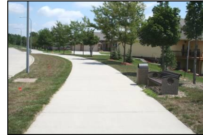
Photo C-42: Lakewood Villages Sidewalk
