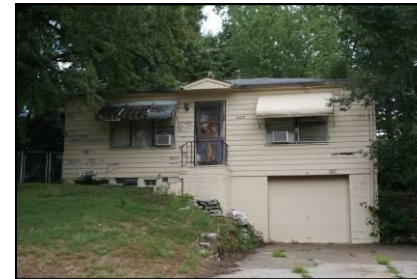
Photo C-35: Northwest District House
