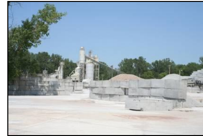
Photo 3-7: The Bellevue Industrial Yard
