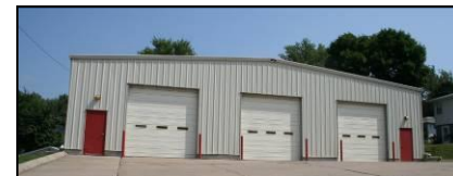
Photo B-29: District 2 Station
