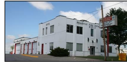
Photo B-30: District 3 Station
