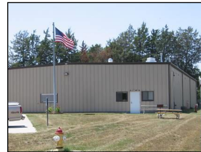
Photo B-40: South Street Shop and Yard
