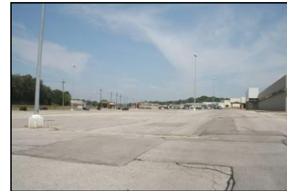
Photo C-23: Large Parking Lots on Fort Crook
