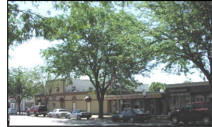
Photo 3-5: The Bellevue Olde Towne Commercial District
