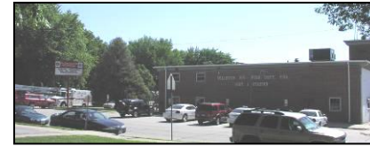
Photo B-27: District 1 Station
