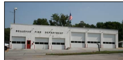
Photo B-28: District 2 Station
