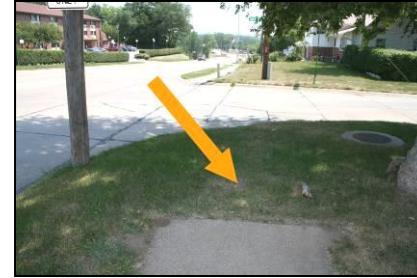
Photo C-5: Sidewalk Abruptly Ends
