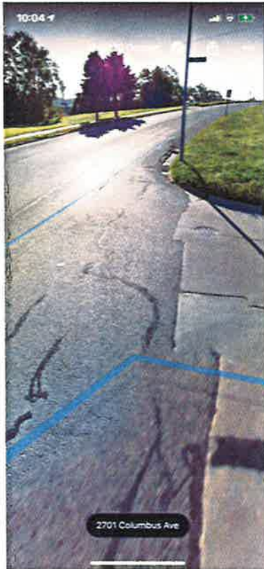
Image #5: View from intersection of Columbus Avenue and Nebraska Drive looking South, as if driver turning right. This image somewhat shows how cars parked along lower Nebraska Drive will make it extremely dangerous and impossible for drivers to see around and turn left.
