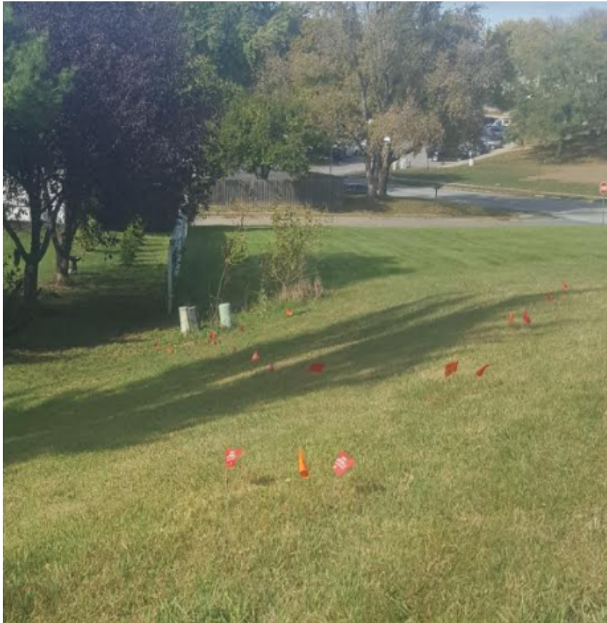
Image 3: This picture shows the underground wiring marked by diggers hotline (811) within the hill on the north side of property Lot 13. – taken 10/17/2020
