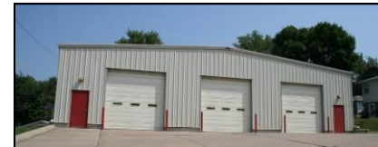
Photo B-36: District 2 Station
