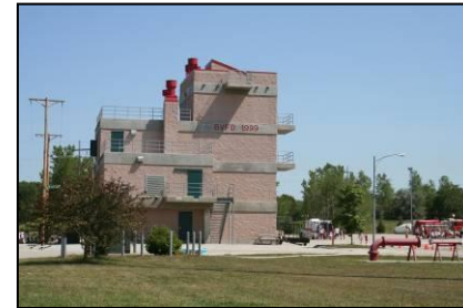
Photo B-39: Fire Training Facility
