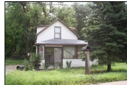
Photo C-37: Northwest District House
