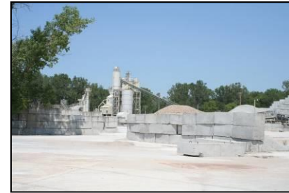
Photo C-33: Concrete Industrial Facility
