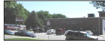
Photo B-34: District 1 Station
