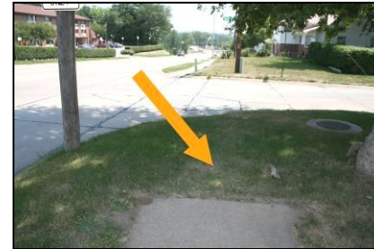
Photo C-5: Sidewalk Abruptly Ends
