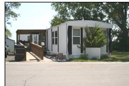
Photo 3-2: A Bellevue Mobile-Home Residence
