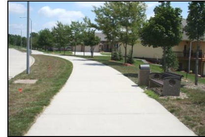
Photo C-43: Lakewood Villages Sidewalk
