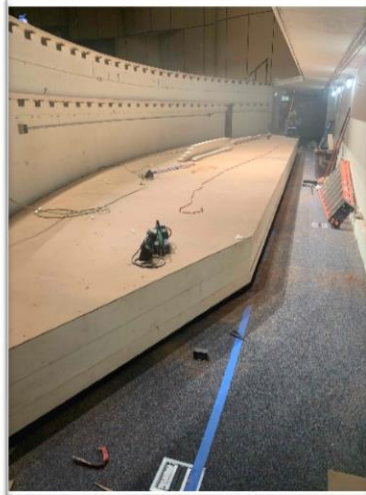
Phase 2: Wood Substrate over lift platform, sides, and ledgers
