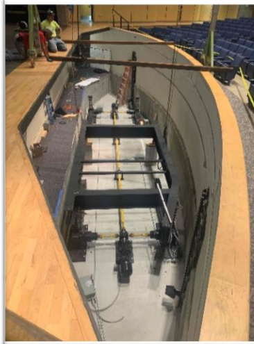
Phase I: Electrical rough-in, rigid chain columns, motors, guide rails installation underway
