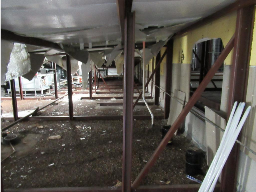
Photo 7 – Metal roof overbuild framing
