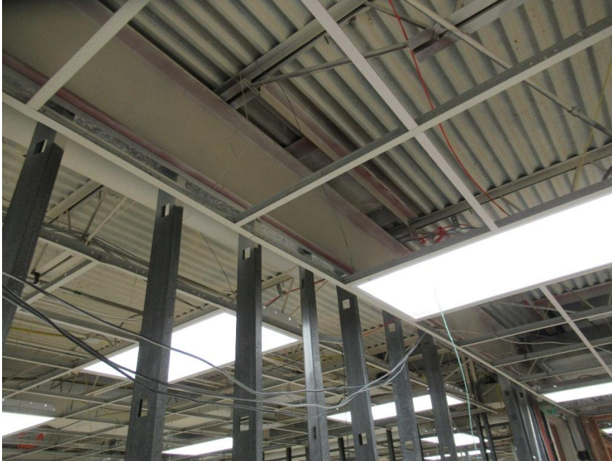
Photo 3 – Original roof steel beam and joist framing
