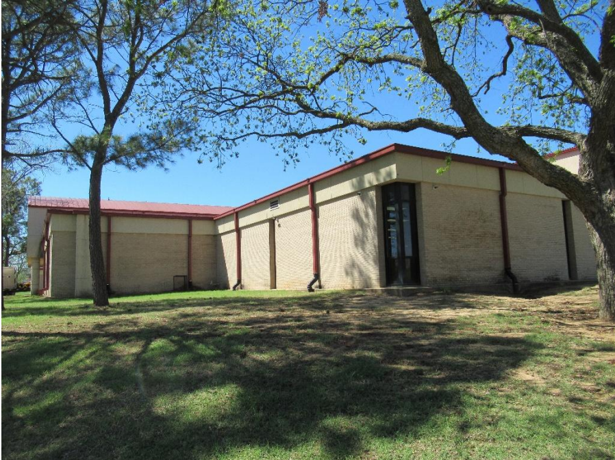
Photo 5 – Exterior brick masonry
