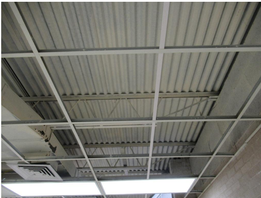
Photo 2 - Original roof metal deck and steel joist framing
