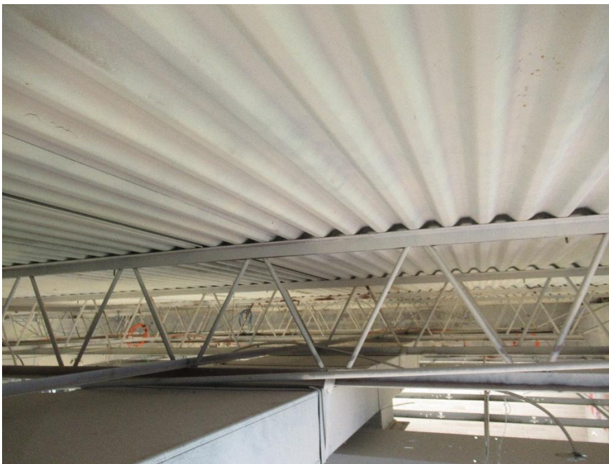
Photo 10 - Original roof steel joist framing - no indications of damage
