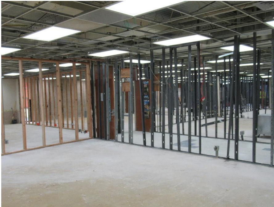
Photo 1 - Overall view of roof framing and interior partition walls
