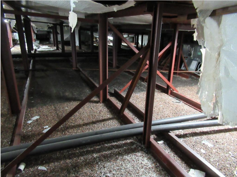
Photo 6 – Metal roof overbuild framing
