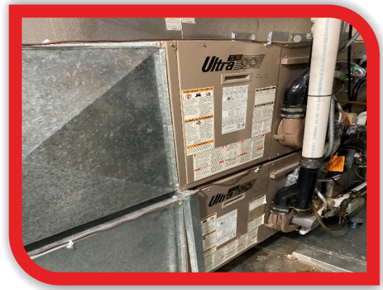
High School Mechanical Roof
