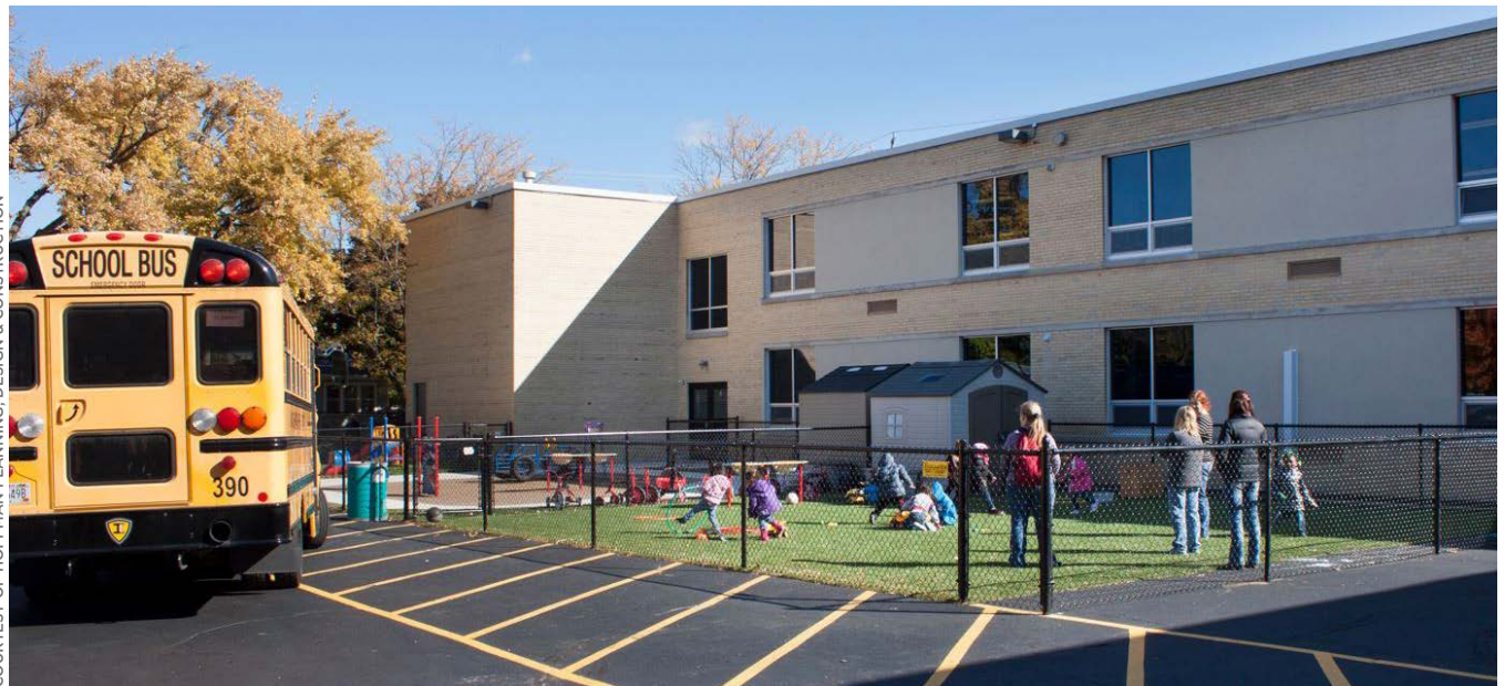
COURTESY OF HOFFMAN PLANNING, DESIGN & CONSTRUCTION
