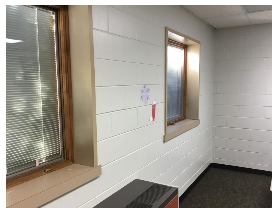
2 EXISTING WINDOW PHOTOS 12" = 1'-0"
