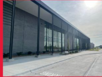
New Springfield Elementary School location, opened in 2022
