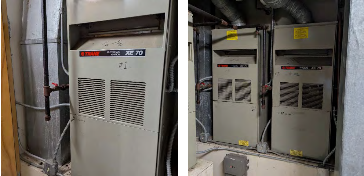
Figure 7. First floor vertical air handlers
