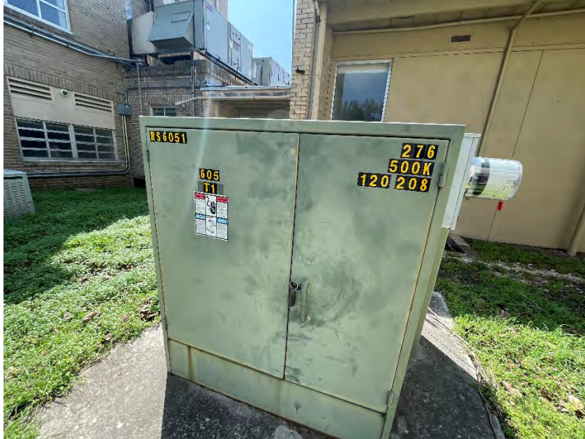
Figure 16. Utility transformer
