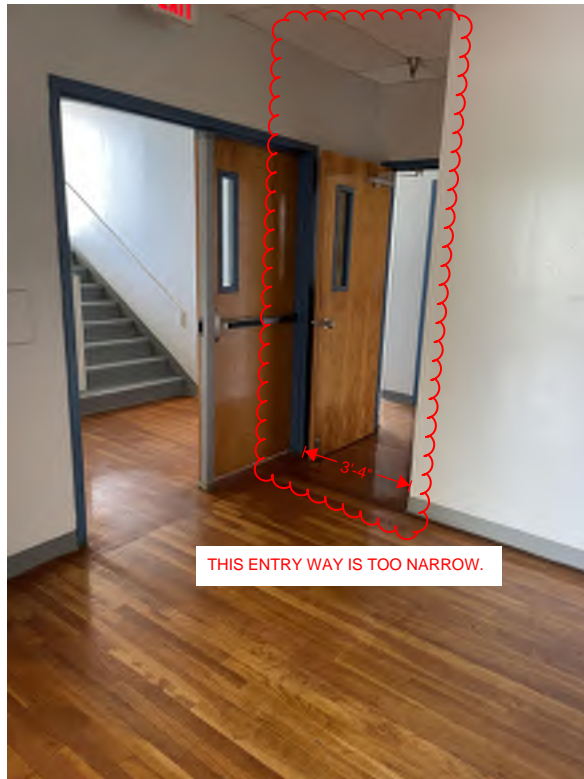
Figure 28: Third Floor Level stairway
