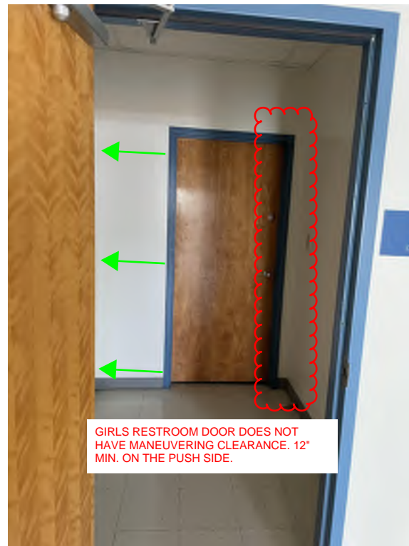
Figure 14: First Floor Basement Girls Restroom
