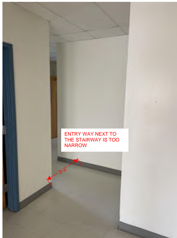
Figure 18: First Floor Basement Stairway
