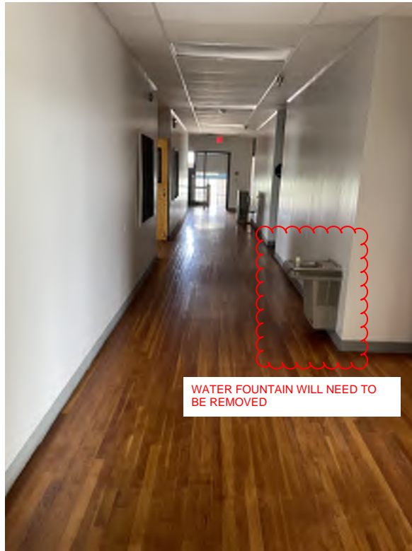
Figure 25: Third Floor Level Corridor
