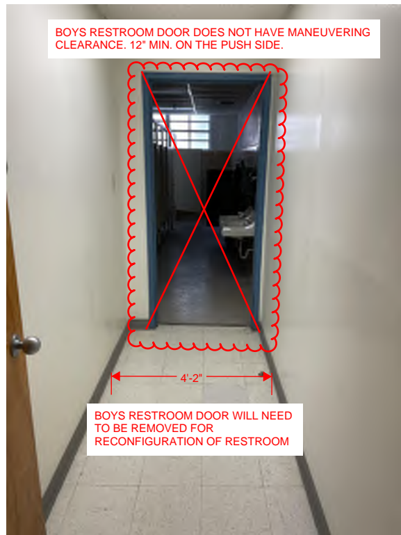
Figure 16: First Floor Basement Boys Restroom
