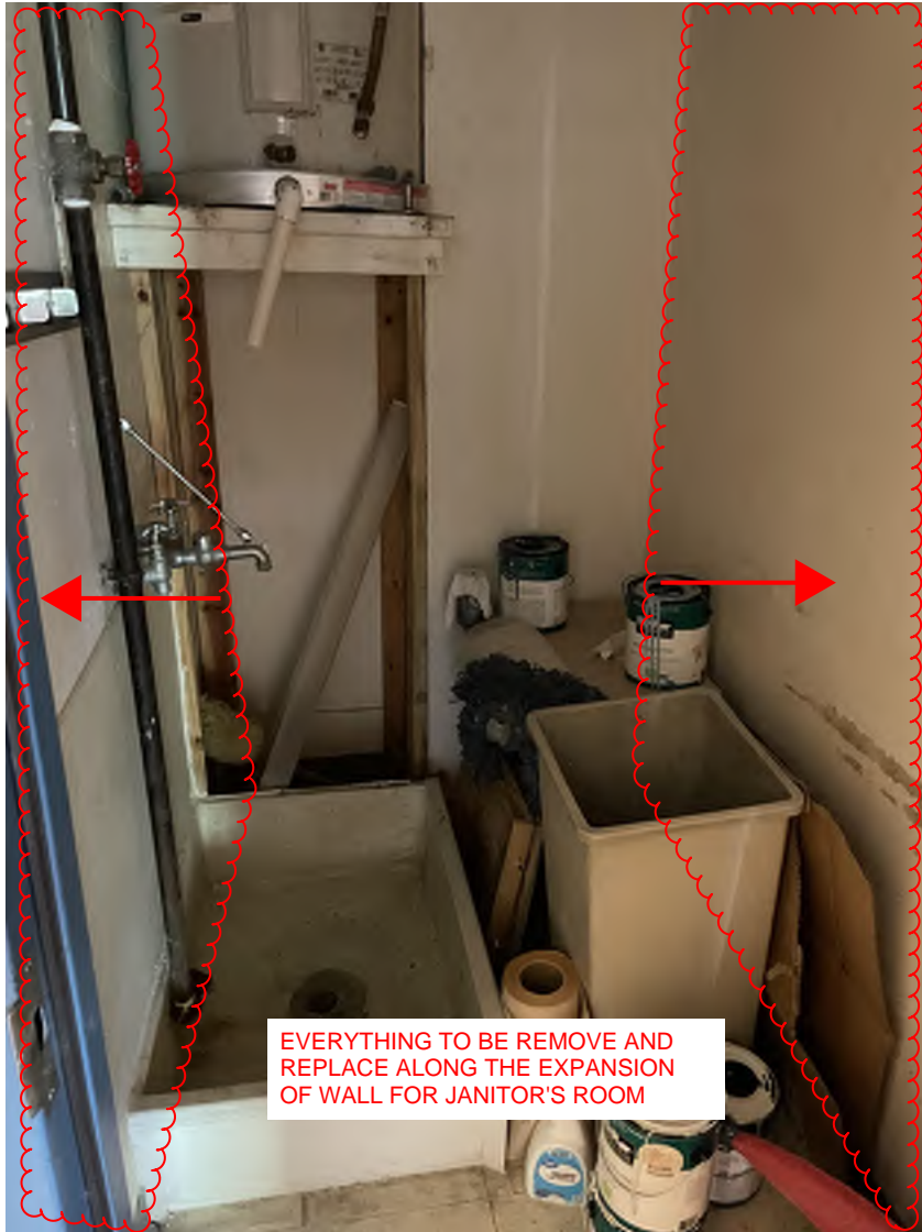
Figure 29: Third Floor Level Janitor's room
