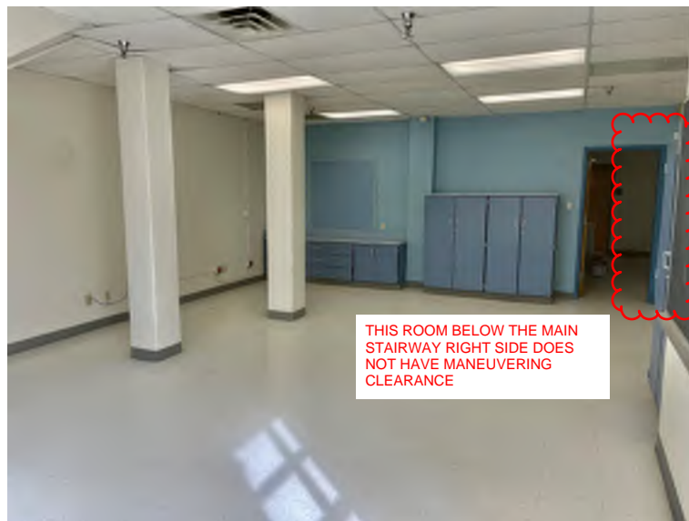
Figure 12: First Floor Basement interior doors
