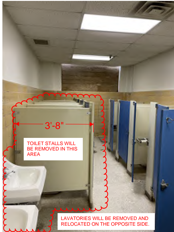
Figure 15: First Floor Basement Girls Restroom
