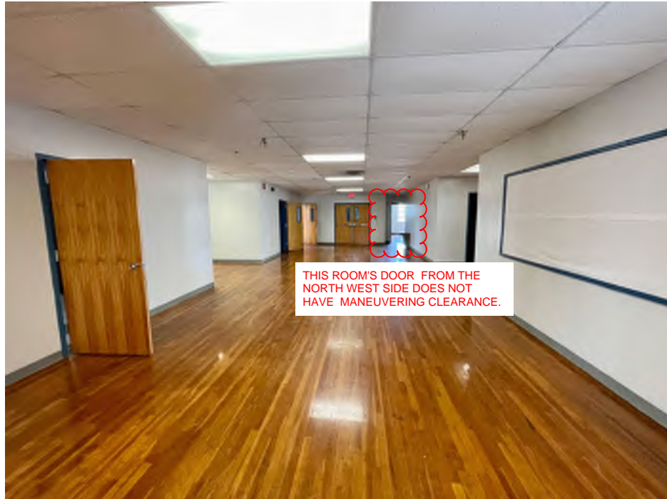
Figure 21: Second Floor Main Level Lobby
