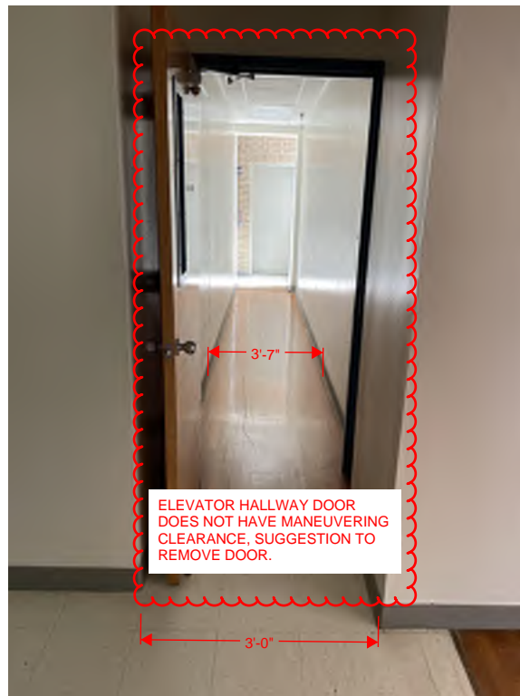
Figure 10: First Floor Basement Elevator Hallway
