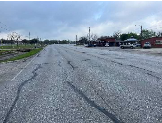
Looking southwest along US Highway 90, subject on left
