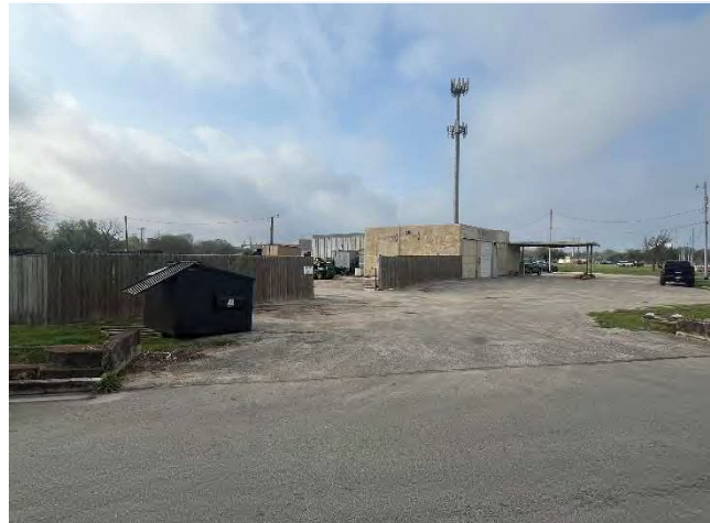
Looking south at whole property from Hummingbird Ln
