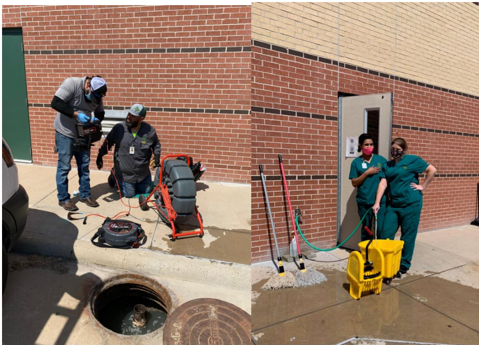
Top left, Carlos Leal and David Serna use the drum machine with camera to find out what is clogging the lines outside of RFMS Cafeteria. While there, I had 2 of the cafeteria ladies that really wanted to be famous and be in my report so I granted their wish. Sasha Guzman and Courtney Eady are representing the cafeteria staff across our district in this picture. Quite often the cafeteria staff go unrecognized and I want to point out how vital they are to the success of our students. Thanks to the cafeteria staff and especially for the good nature of these two ladies posing for the picture.
