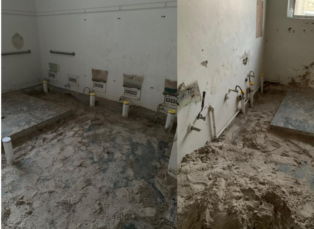
Above you can see where all new plumbing was added to the ladies restroom inside the what will be administration offices.
