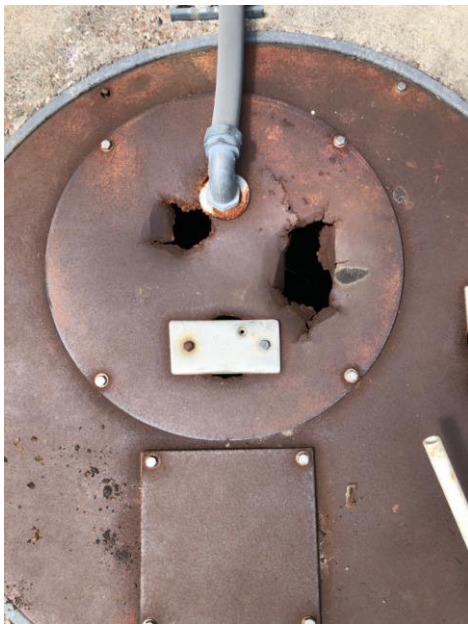
So the above lift station for the sewer system that services the CATE Building needed a new top. The picture on the left was the original and the right is what it looks like now.
