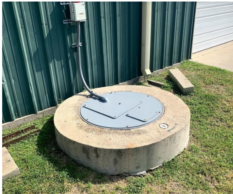
So the above lift station for the sewer system that services the CATE Building needed a new top. The picture on the left was the original and the right is what it looks like now.
