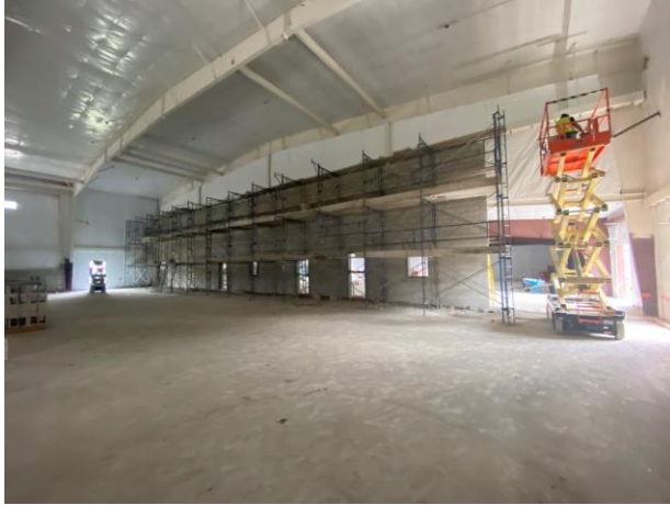
CMU "Concrete Masonry Unit" is still going up but this is the separating wall between the court side and the dressing room side taken from the court side.
