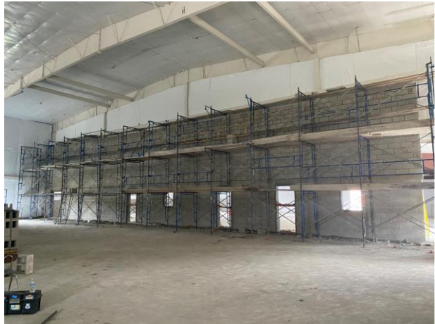
CMU "Concrete Masonry Unit" is still going up but this is the separating wall between the court side and the dressing room side taken from the court side.
