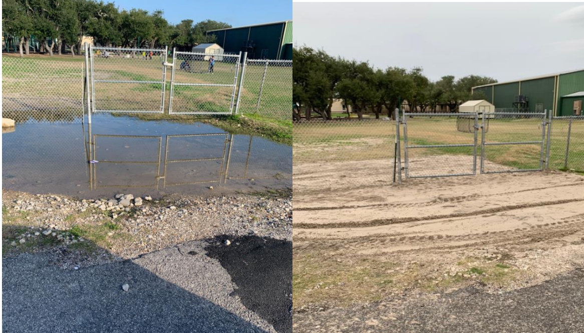
Above left, you can see where there was a very low spot at the back gate of FLC playground. We brought in some fill dirt and spread it around that area to make it level.
