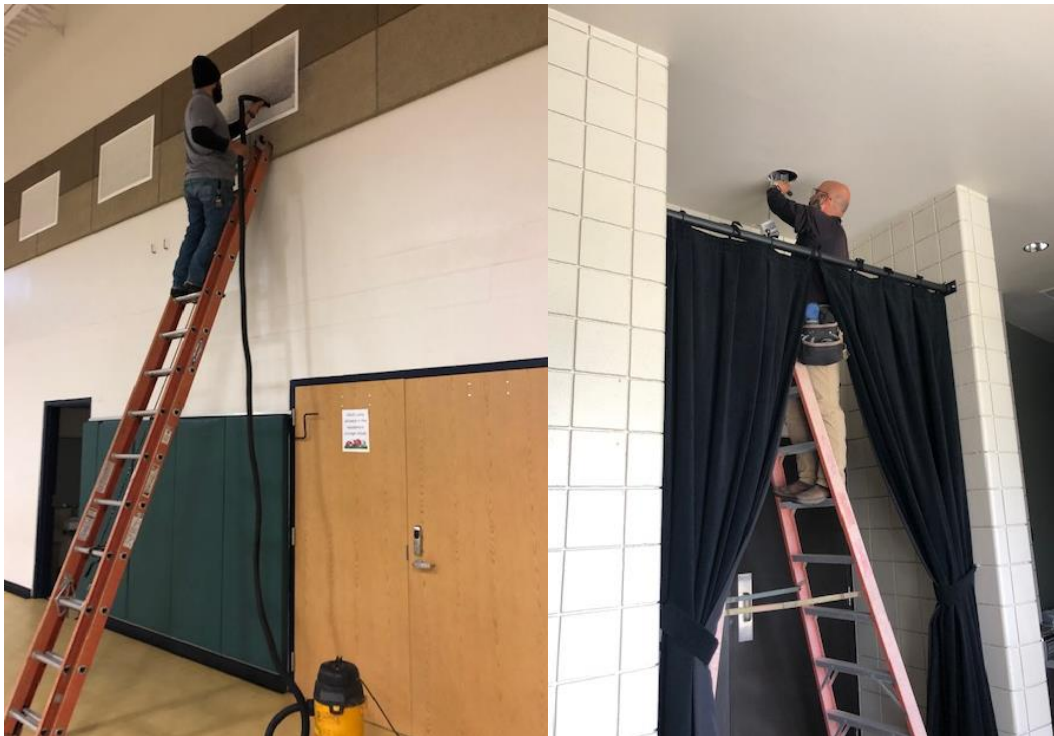
Above left, Carlos Leal cleans the AC return vents out at LOLC gym. Top right, Dwayne Solis repairs a light fixture in the Martha Luigi Auditorium.
