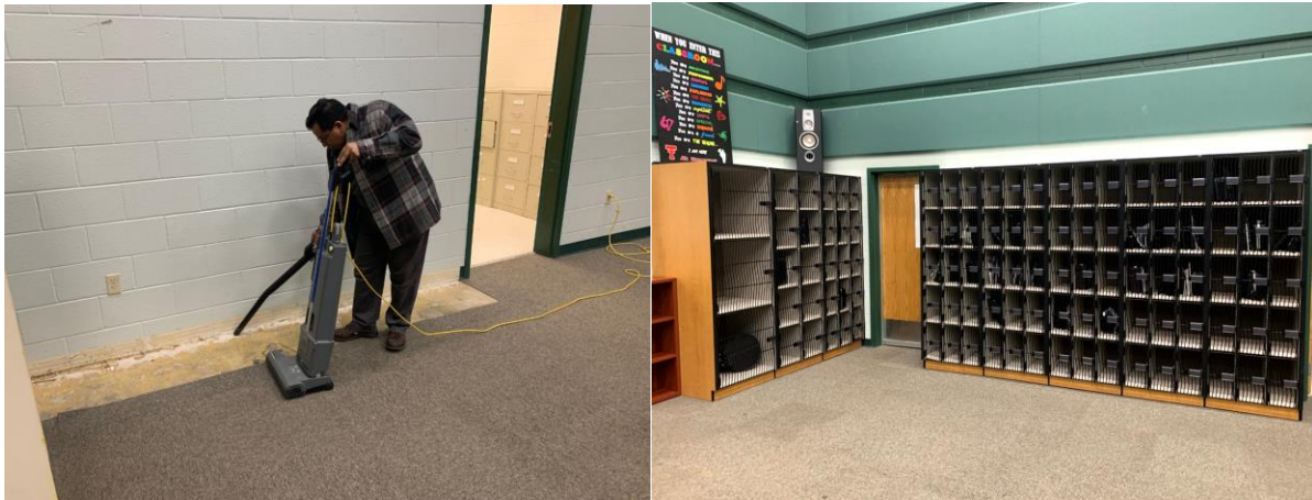
Lead custodian, Mark Castro cleaning the area before the installation of the new lockers installed in the RFMS Band Hall.
