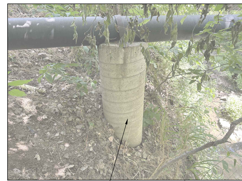
DEMOLISH EXISTING CONCRETE PIPE SUPPORT
