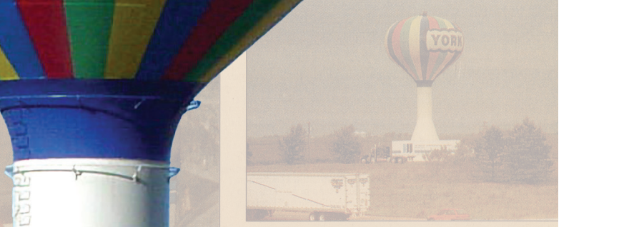
York Public Works employee Dave Becker opened up the valve in the base of the water tower. The new 750,000 gallon water tower will be dedicated during Yorkfest in September, which
