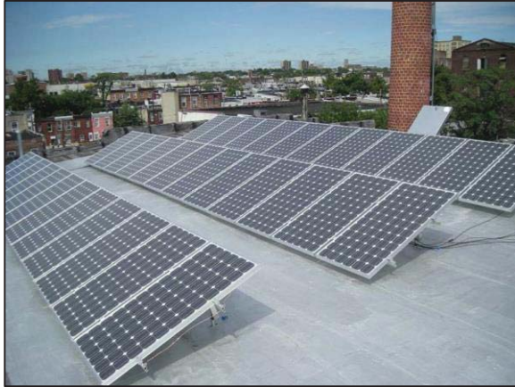
Roof top application of an older building in Philadelphia.
