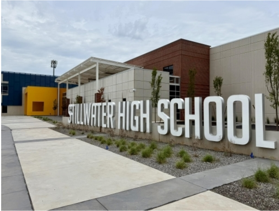
FRONT ENTRY AND DROP-OFF
