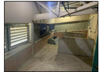
Completely Demoeed N Mezzanine
