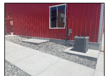
Concrete Pad for New Locker Room Units
