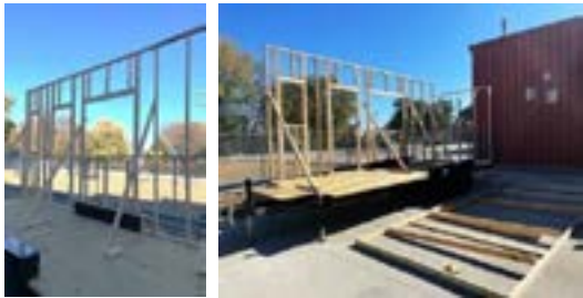
The First Walls
