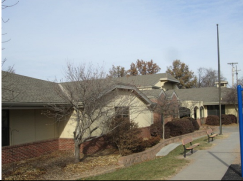
West exterior showing no code required upper roof venting.
