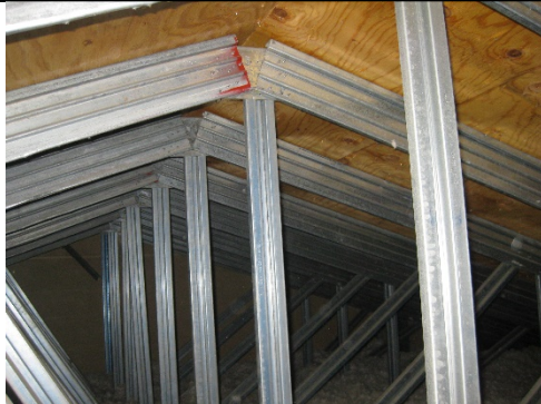
Attic space on South side of building showing no moisture damage.
