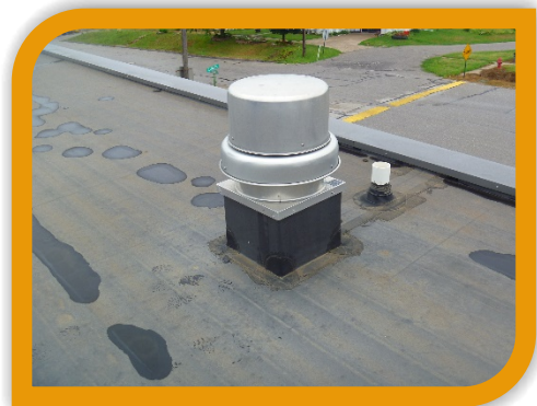
Powered Exhaust Fan
