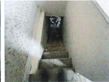
Stairs to Below Grade
