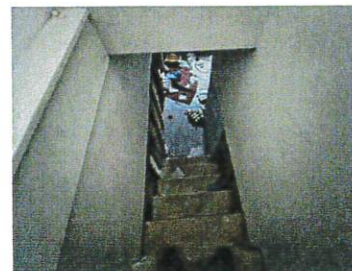
Stairs to Below Grade
