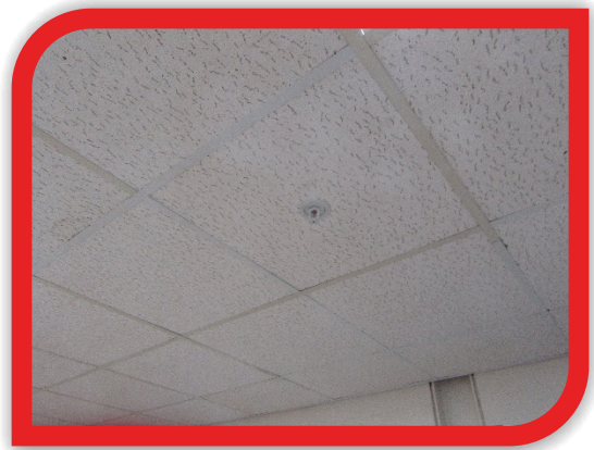
Elementary Fire Sprinkler
