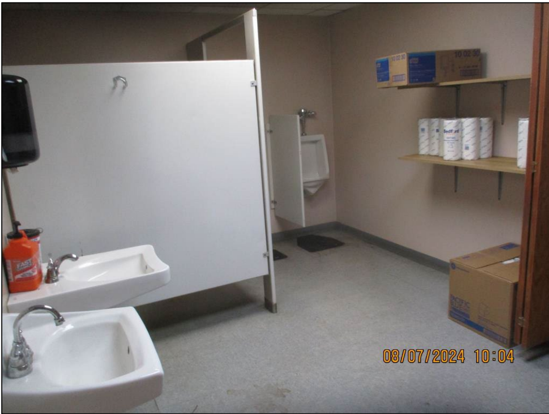
31001 Building- Men's Bathroom
