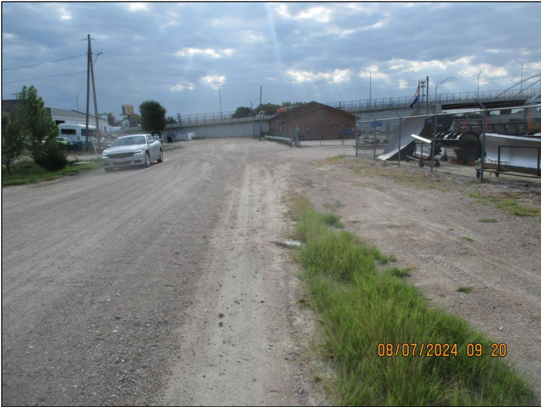
Street Scene- 12th Street: West to East
