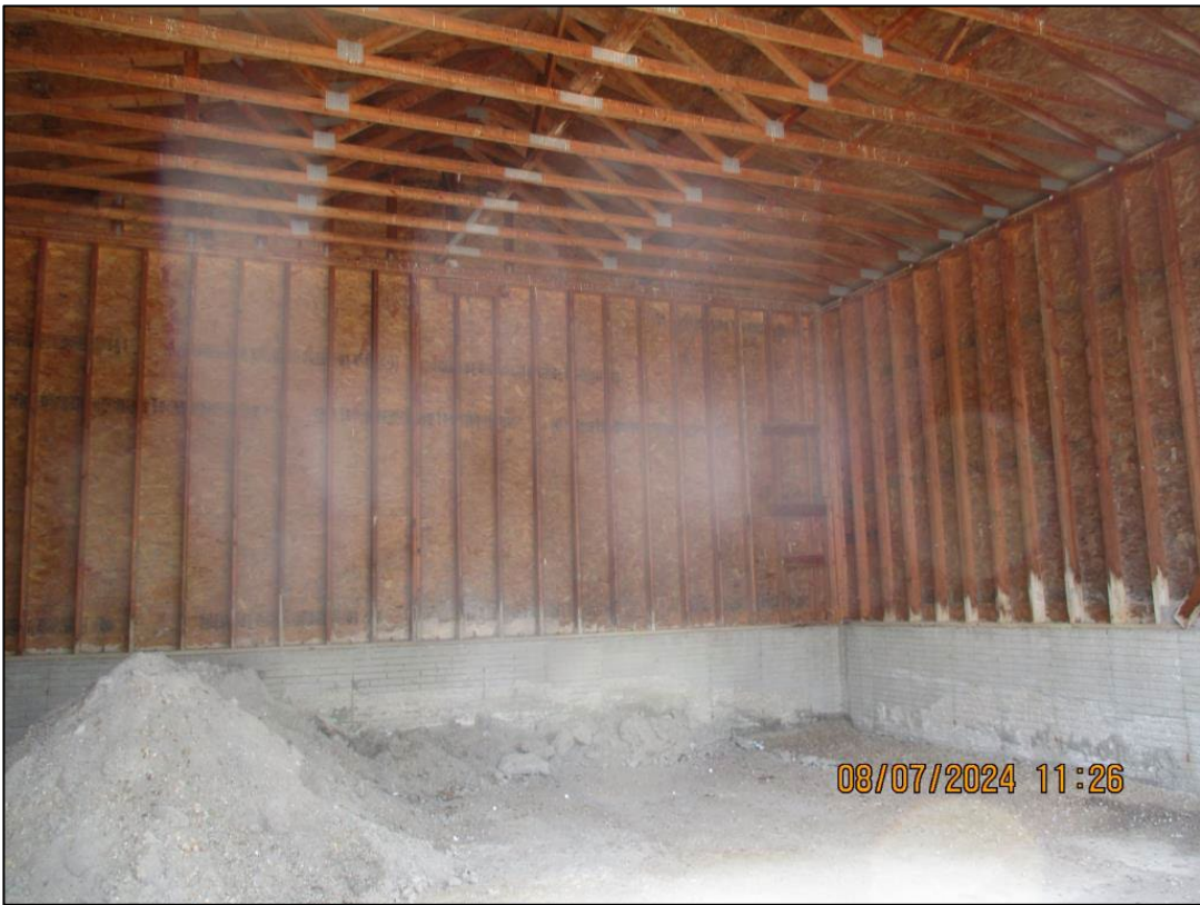
No Bldg #- Miscellaneous Storage Building- Interior
