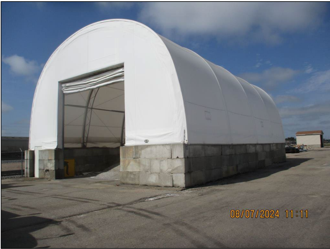
Building 31011- Fabric Building
