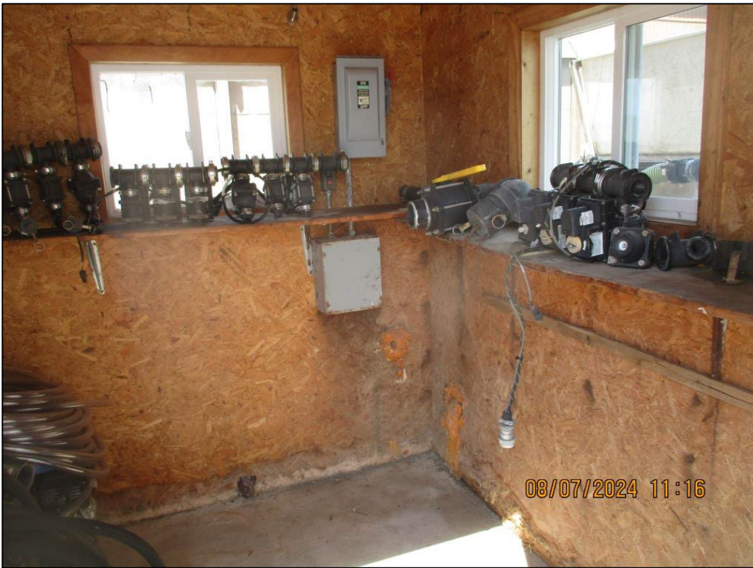
No Bldg #- Misc. Storage Building b- Interior
