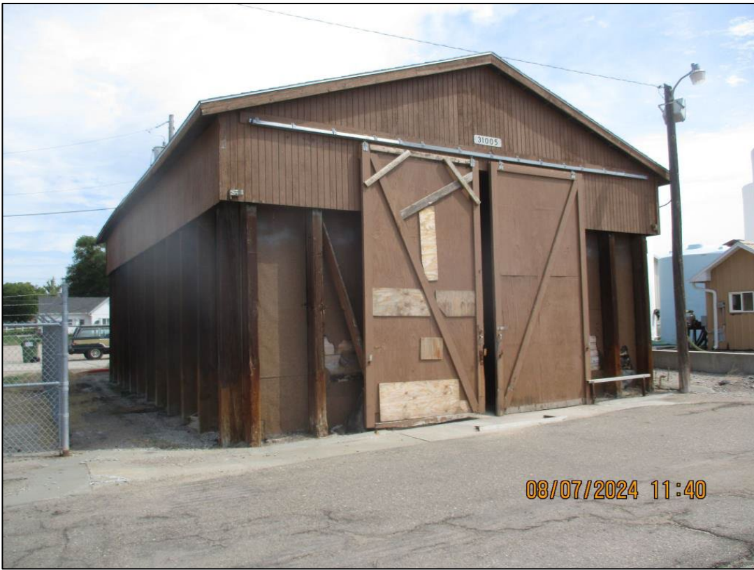
31005 Building- Bulk Salt Storage
