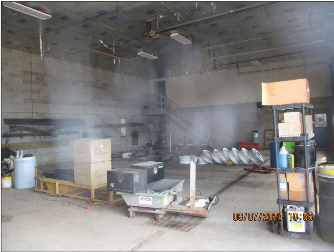
31009 Building- Shop Area
