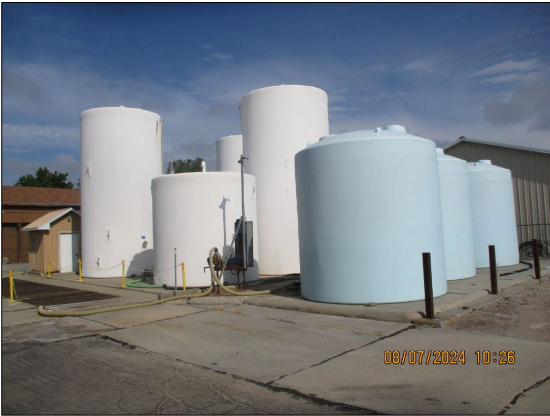
No Bldg # -Miscellaneous Storage Building b
