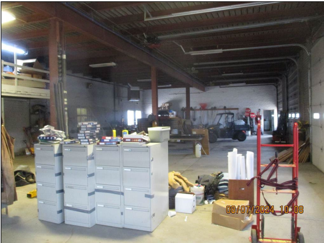
31001 Building- Shop Area a
