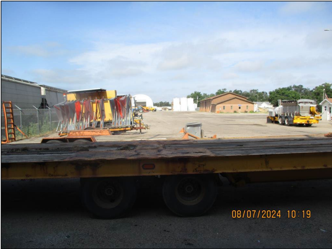
Site- Southeast PL to the West
