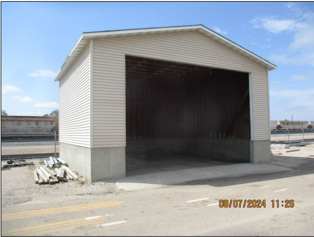
No Bldg #- Miscellaneous Storage Building
