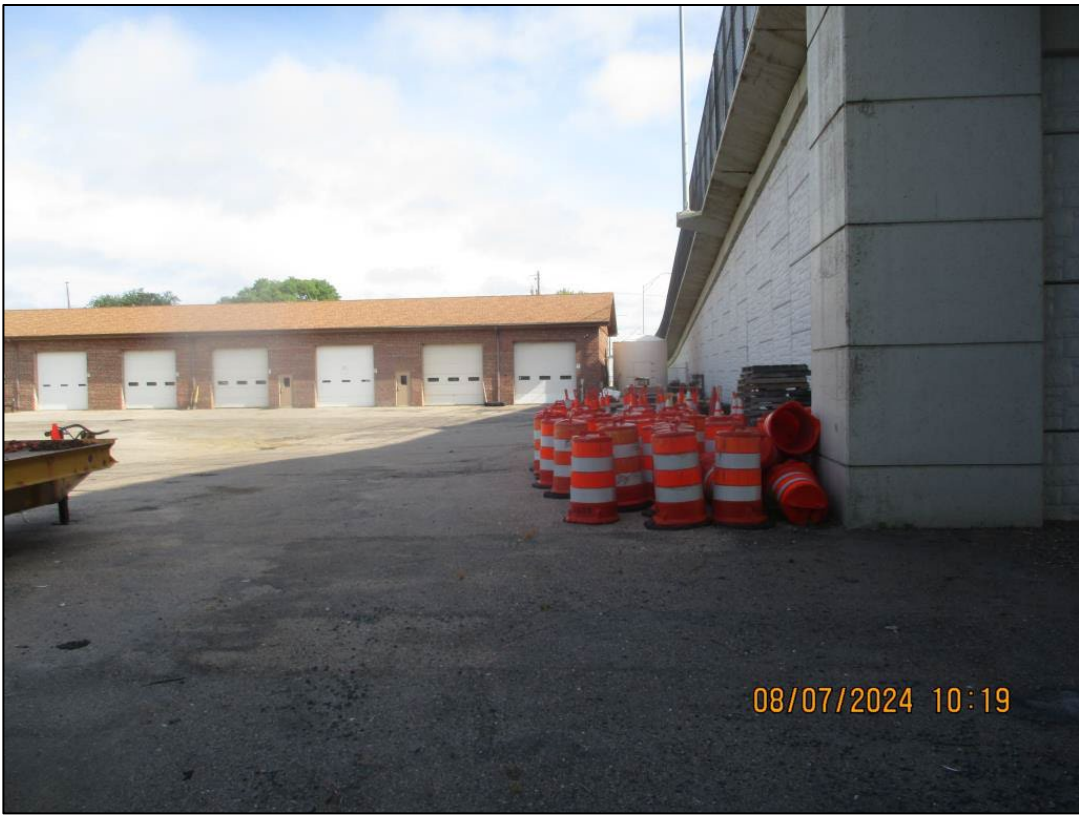
Site- Southeast PL to the North
