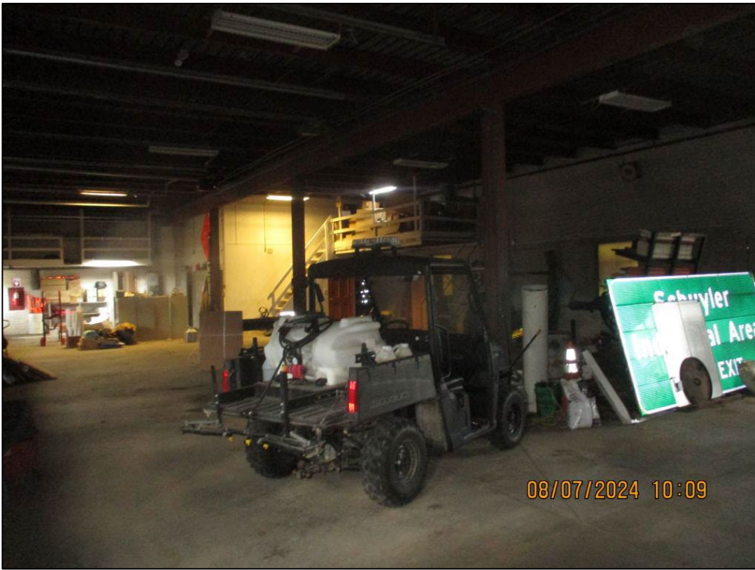
31001 Building- Shop Area a
