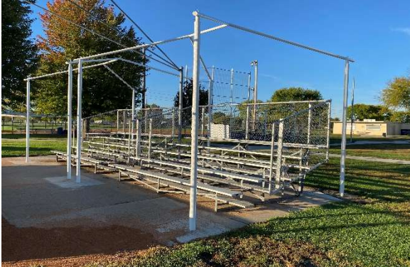
FIGURE 2.12 // EXISTING COVERED BLEACHERS
