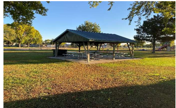
FIGURE 2.07 // EXISTING PLAYGROUND SHELTER (WEST)
