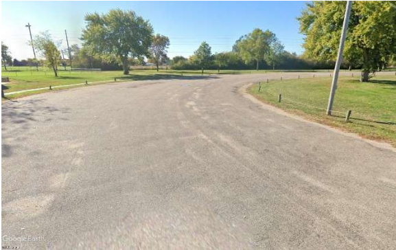
FIGURE 2.13 // EXISTING PARKING LOT
