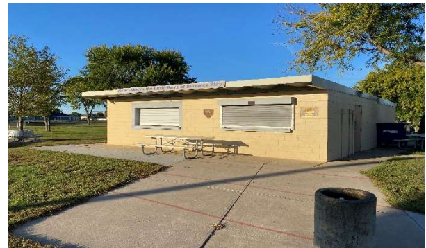
FIGURE 2.08 // EXISTING CONCESSION BUILDING
