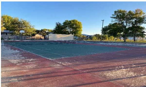
FIGURE 2.04 // EXISTING TENNIS COURT
